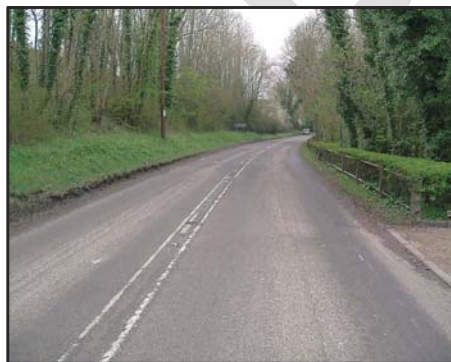
Worn road markings (WEAR)
