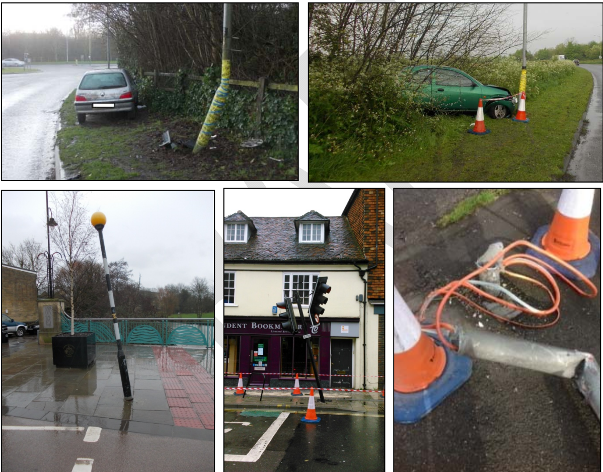
Damaged electrical installations and equipment (LIGH)
